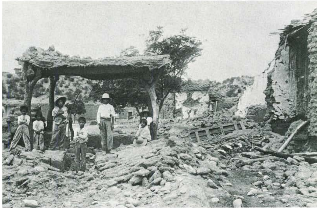
Figure 14. In writing about the destruction at Bavispe, Goodfellow stated, "The remains of the building with the four corner posts standing are those of an exceptionally built one; and a very lucky exception it was in this case, for it saved the lives of four persons who were in it at the time." (4) The original of the photo shown was taken by C. S. Fly. Presumably, the building referenced above is the same as those remains appearing in the photo. Photo courtesy of the Arizona Historical Society.
